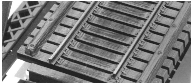
CLOSE UP OF THE-SPIKING DETAIL
