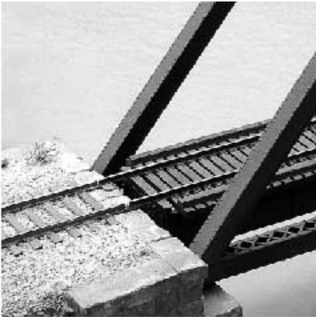
PHOTO SHOWING EASY SET--IN / LIFT-OFF USING MODIFIED RAIL JOINERS
