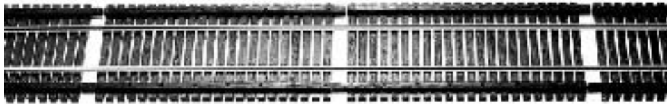
RAIL AND TIE ASSEMBLY SHOWING GAPS
